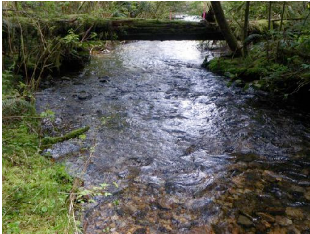
Site 3. – Cedar cross log to be cut, dropped into creek and pinned with rebar to create a sill log.
