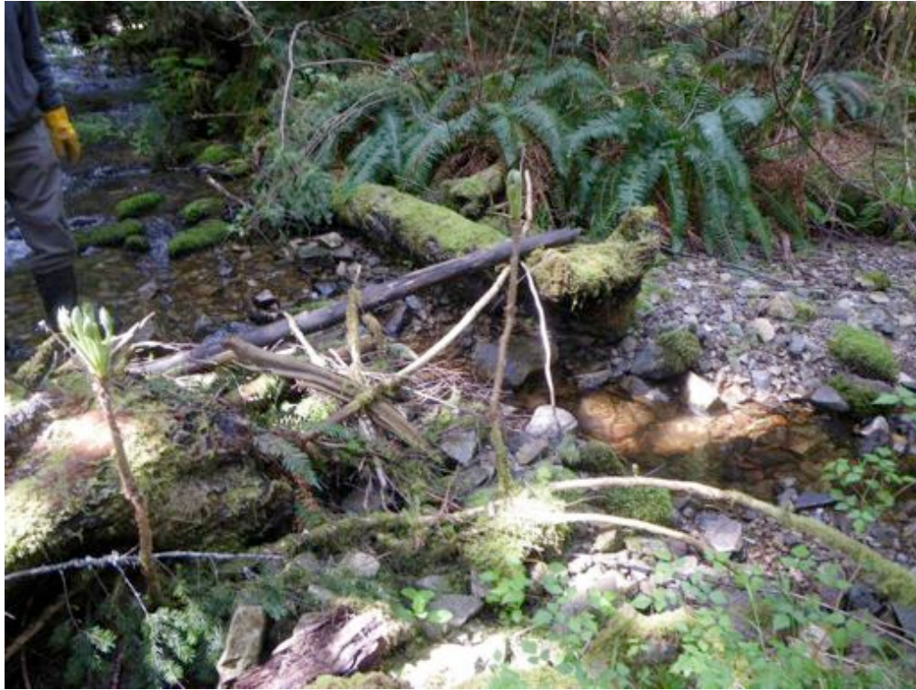
Site 9. – Blocked entrance to the westerly side channel. Stream is to the left. Rock is to be removed from the inlet and used to construct a deflector berm slightly upstream. The berm should cause a back eddy in the channel mouth and remove bar gravel from accumulating in the future.
