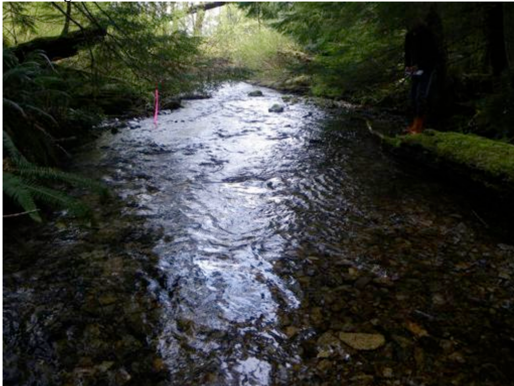
Site 4. – A deflector log is to be installed into the creek (east side) and will extend 2/3 across the creek. The log is to be anchored using 5/16 galv. cable to a stream
